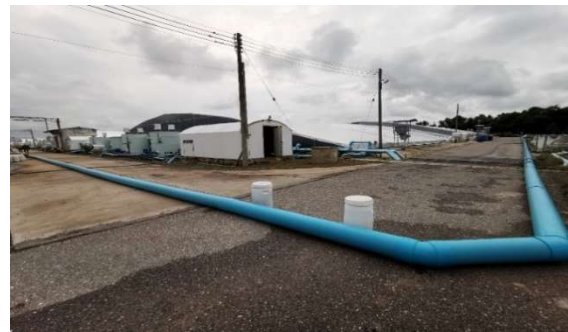
Figure 9 Shows a 10-inch pipe, 360 meters
